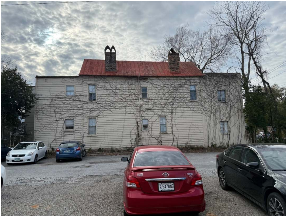
Figure 5. January 30, 2026, image looking approximately west just south of Vanderhorst Street. (photo by M. Scott Harris)
